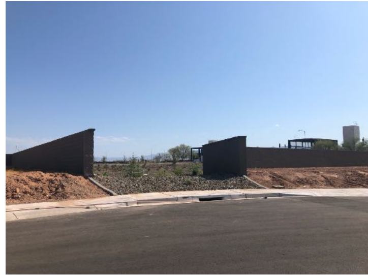
14 – Looking across parcel 19.7 towards the Ironwood Drive entrance on Radiance Avenue.
