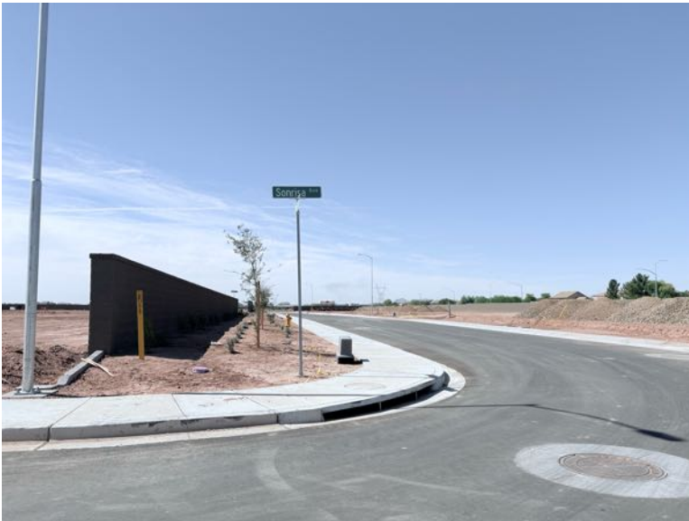
7 – Looking south along Smythe Drive at Sonrisa Avenue.
