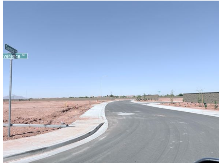
4 – Looking east along Sonrisa Avenue at Reverence Road.
