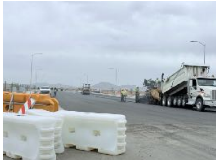
20 – Looking North along Blossom Rock Trail on the east side of Parcel 3A.
