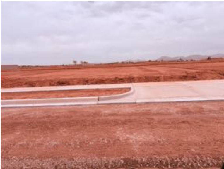
7 – Looking north across Phase 3B.
