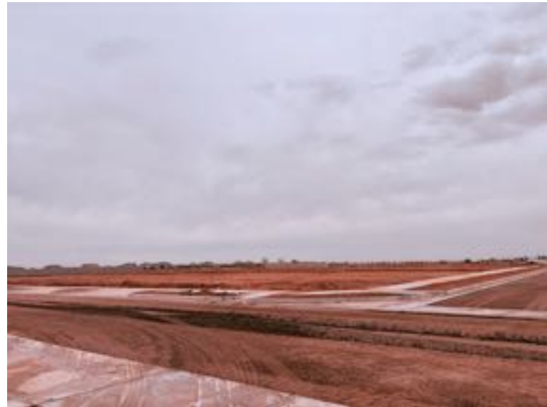
6 – Looking northwest across Phase 3B.
