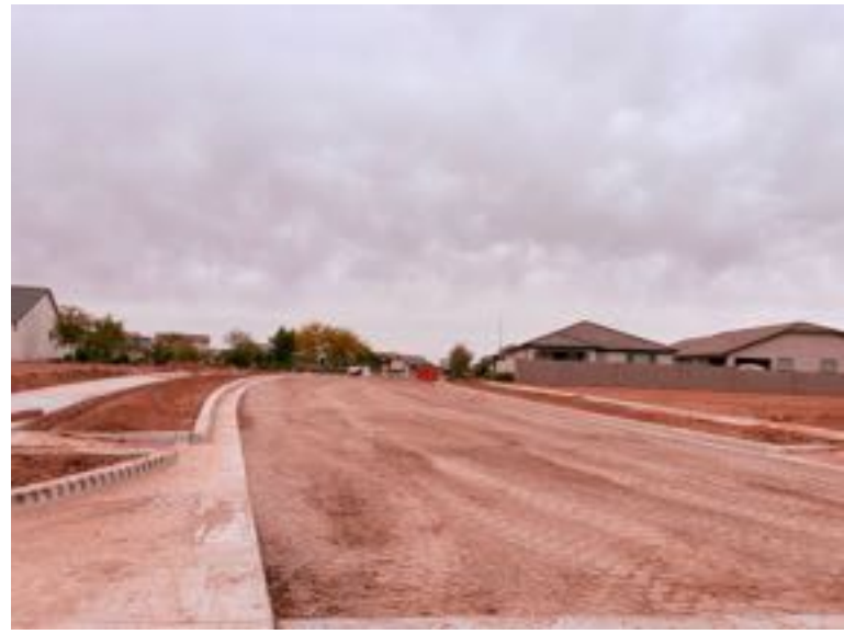
8 – Looking south along Centennial Road at Haynes Way.
