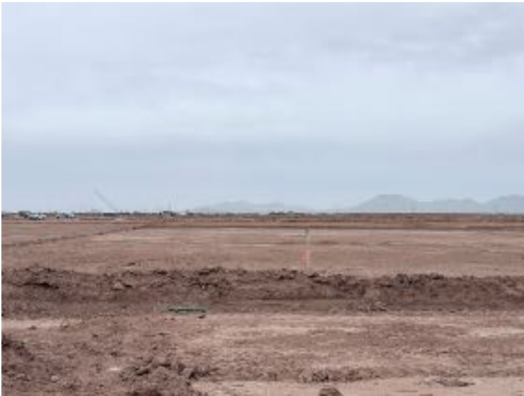
13 – Looking north across Parcel 3A at Barefoot Road.
