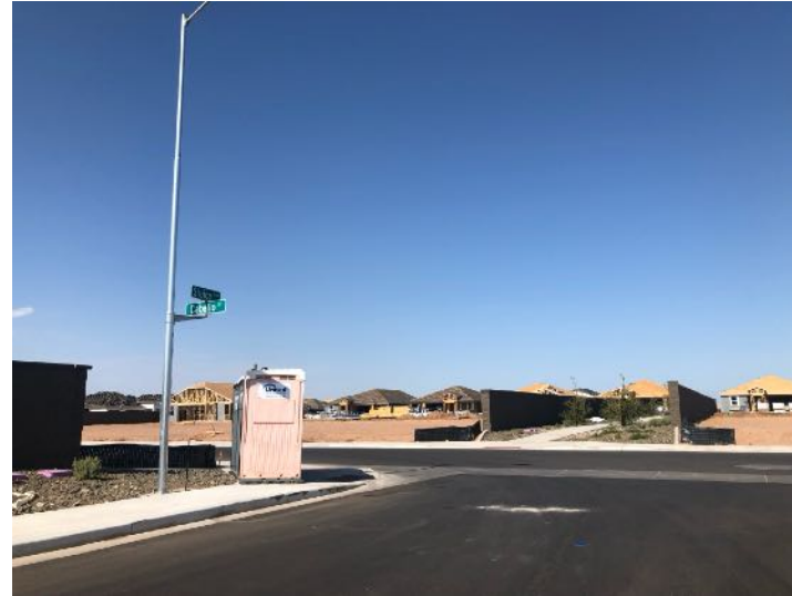
8 – Looking across Caballo Dr. and Sluice Ave. (19.8 & 19.9)
