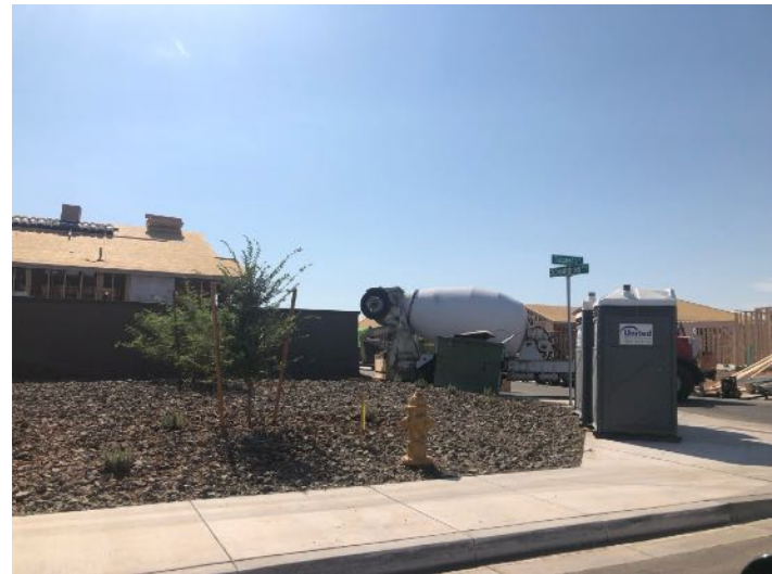
12 – Looking across Spaulding and Saguaro Ave. Parcel 19.6 & 19.7.
