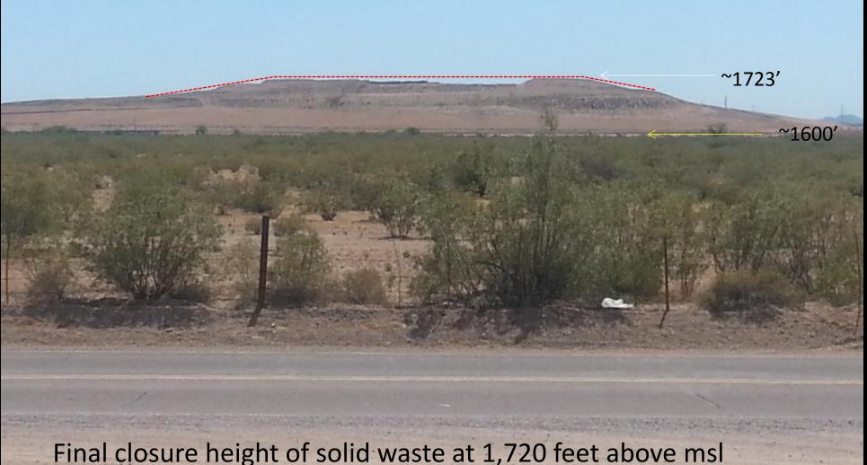
Allow for three feet of cover for total height of 1,723 feet above msl
