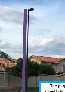
The purple line next to the streetlight depicts the section of the existing streetlight pole that shall be used to calculate the height of the existing pole. The lines are not to scale and are used solely for illustrative purposes.
