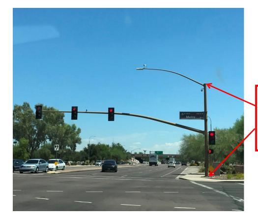
The top and bottom points on a traffic signal pole to calculate the base vertical height of the existing pole
