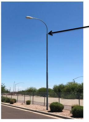
The "connection point" on an existing telescopic style streetlight pole with an integrated luminaire mast arm
